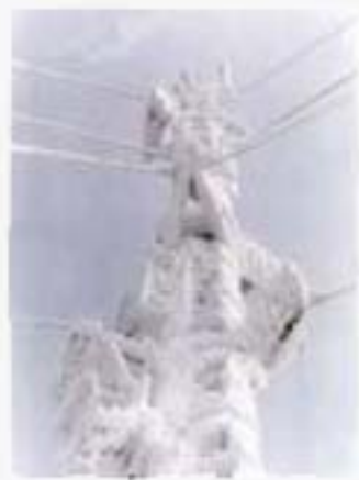
Tower exposed to in-cloud icing
